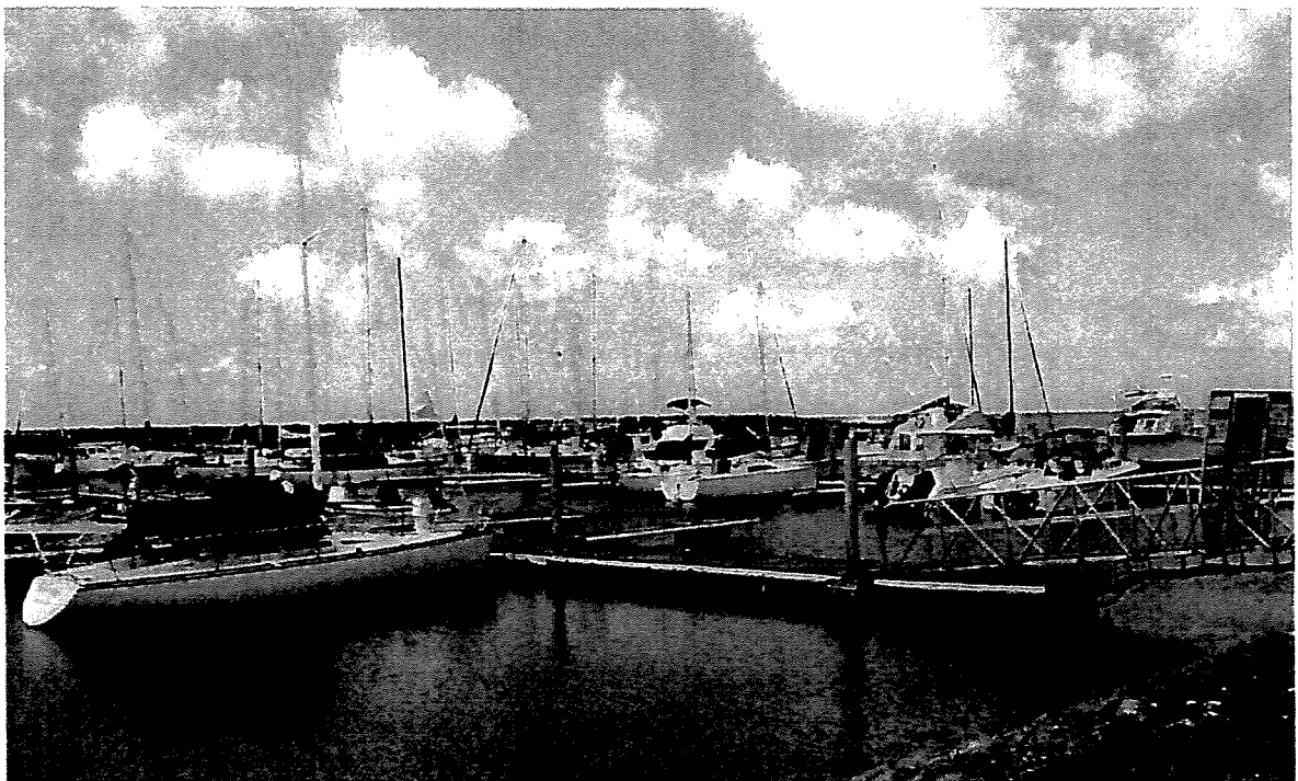
Figure 13: Pier B & C, Agat Marina.
