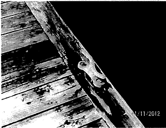
Figure 20: Rotted wood pier.
