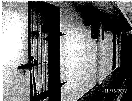
Figure 30: Public toilets at the GPD Office. Note the locks and concrete fractures.
