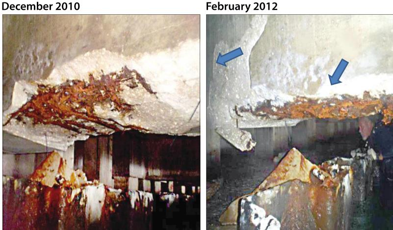
**Bent 9D-E – Progressed damage: spalling**
