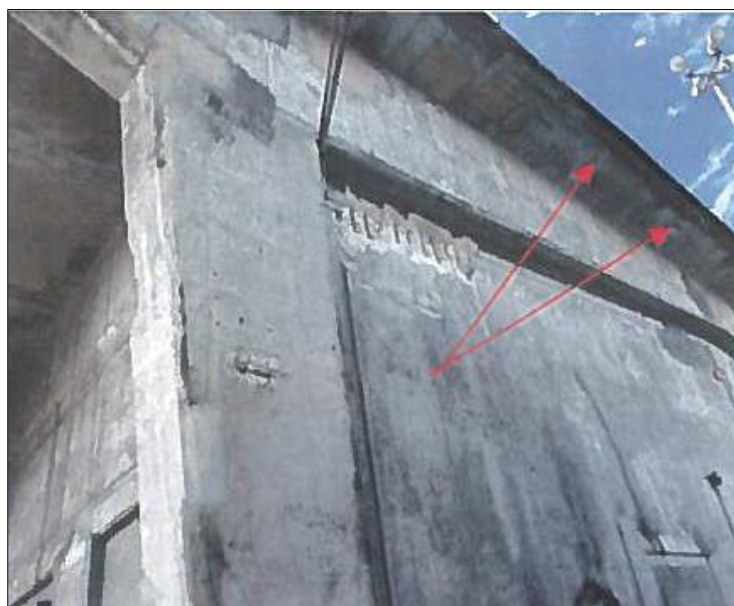
REPAIR SPALLS
