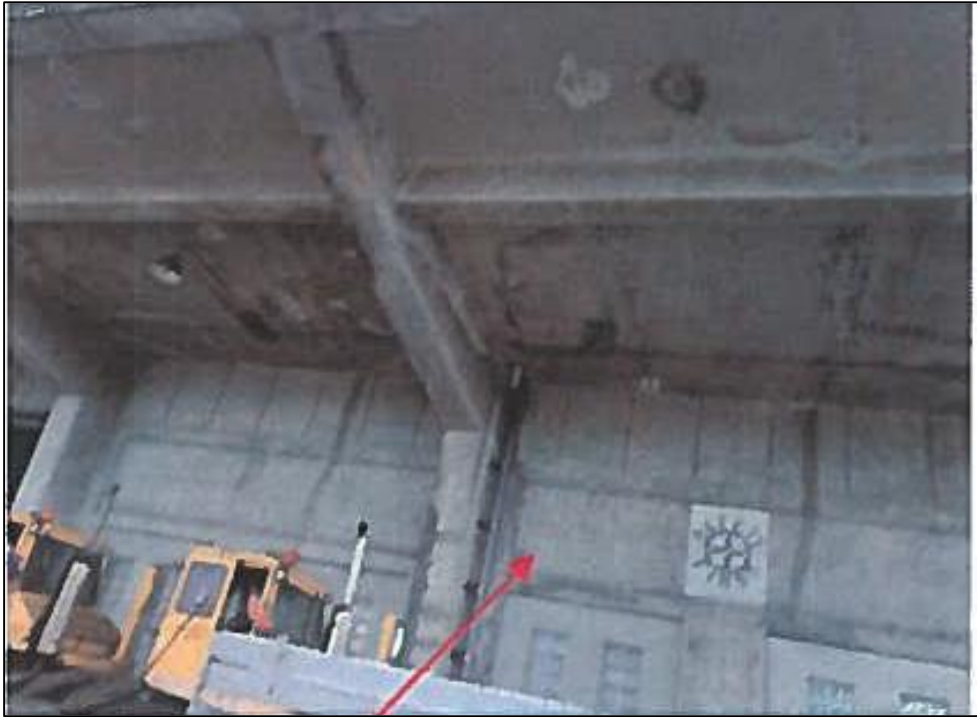
REPAIR SPALL
