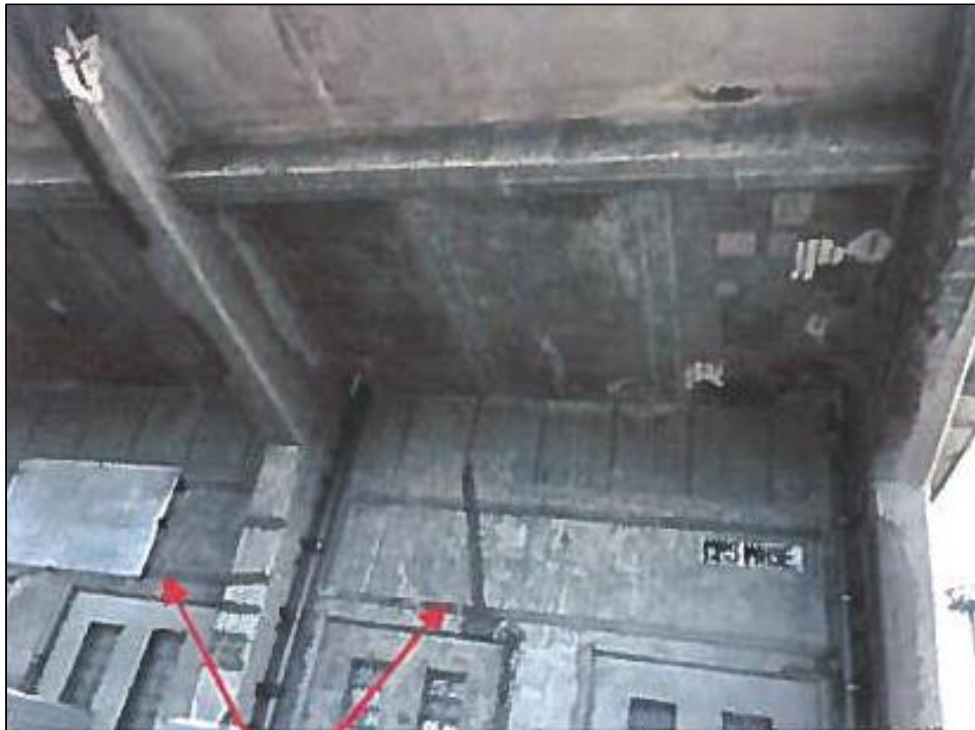
REPAIR SPALLS
