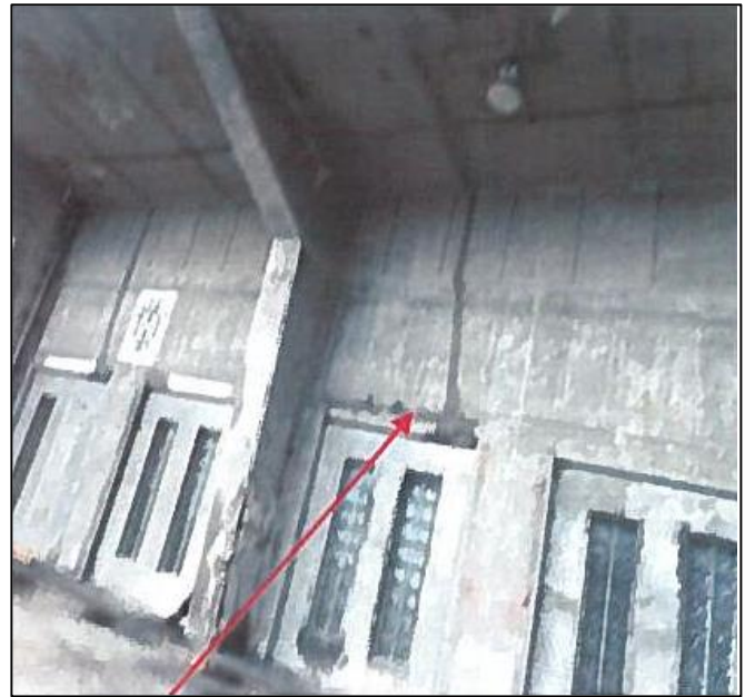
REPAIR SPALLS
