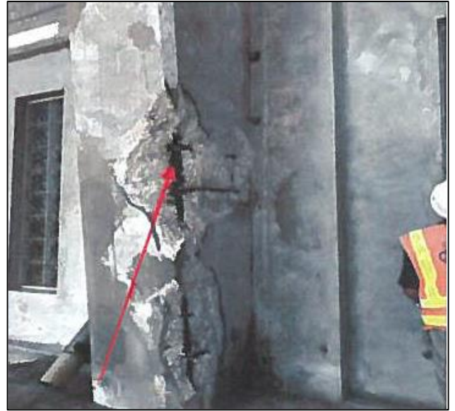
REPAIR SPALLS
