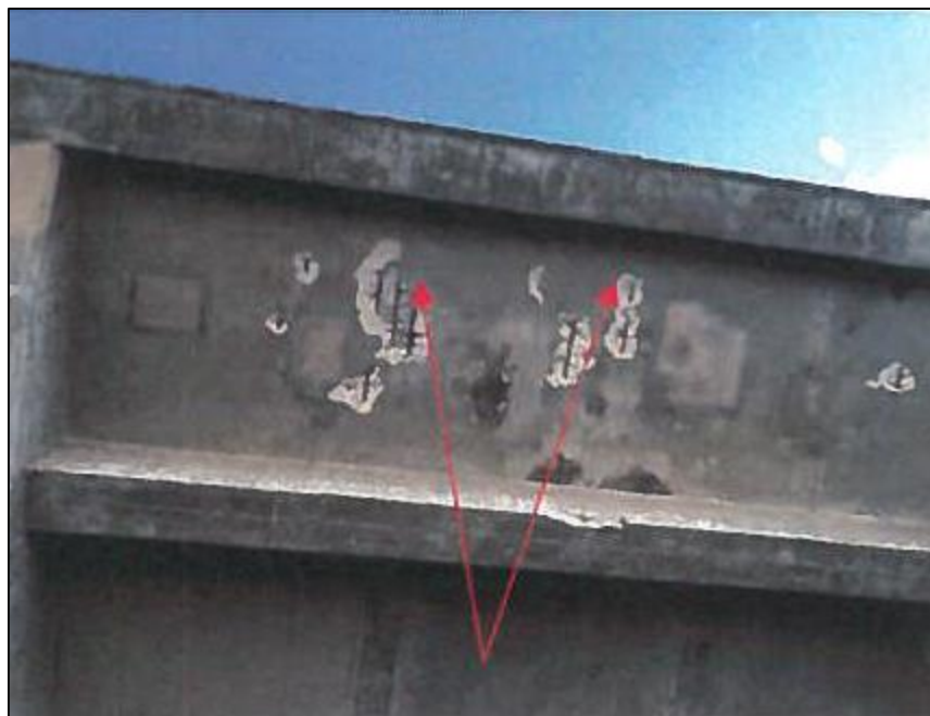
REPAIR SPALLS
