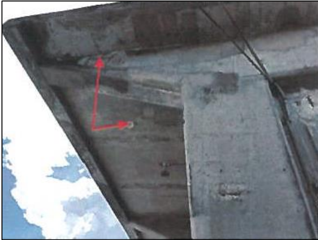
REPAIR SPALLS
