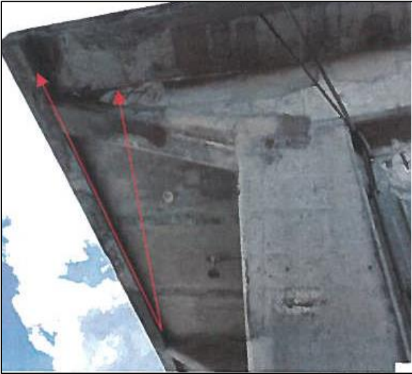
REPAIR SPALLS
