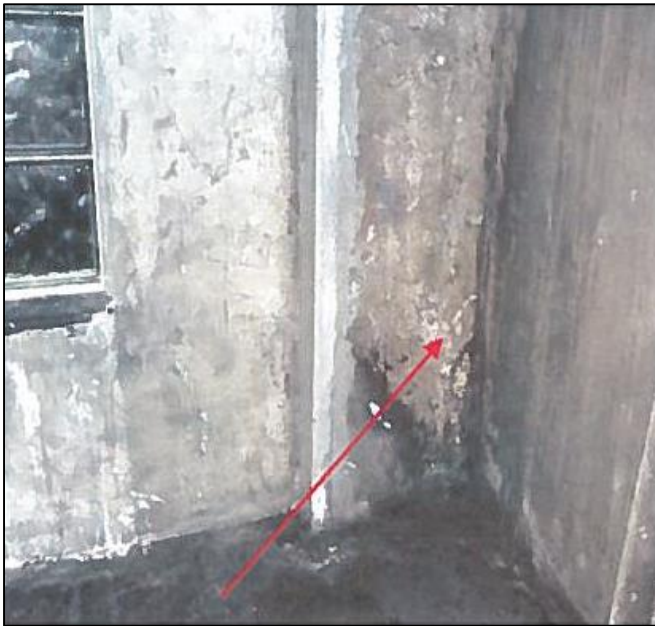
REPAIR SPALLS
