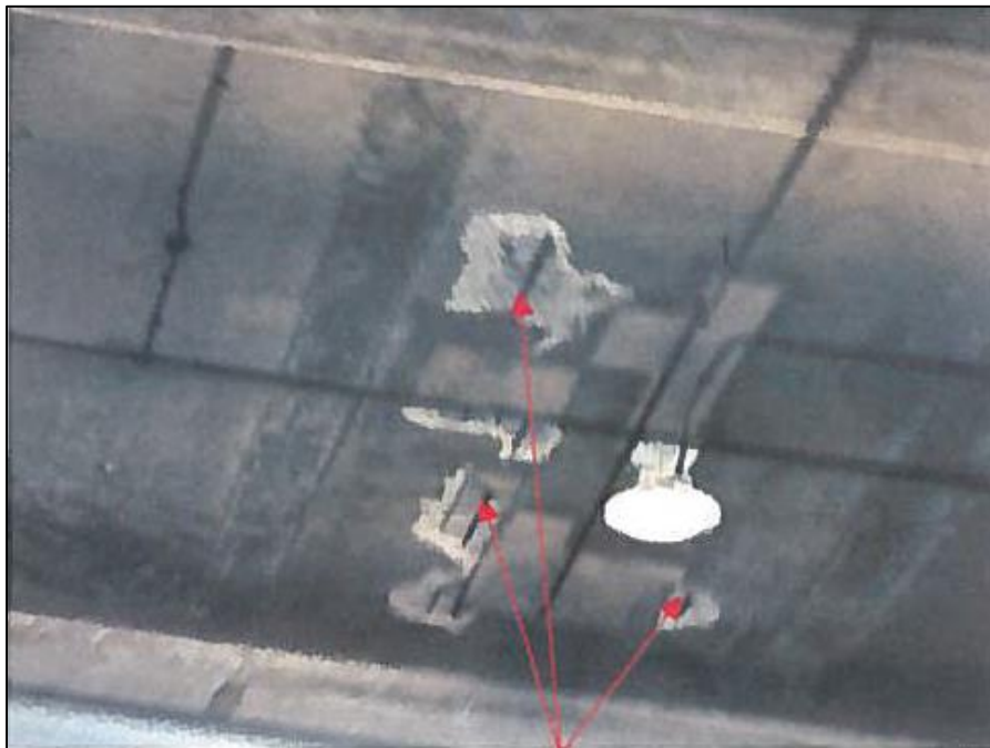
REPAIR SPALLS
