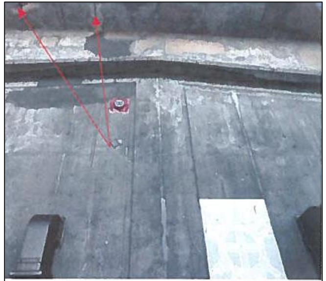
REPAIR SPALLS
