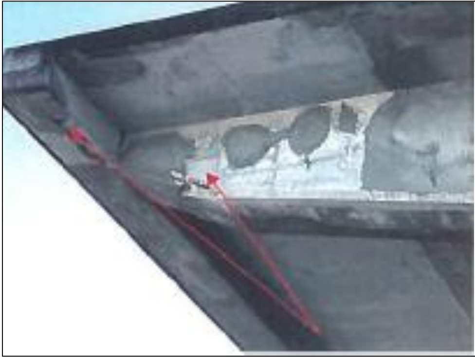
REPAIR SPALLS
