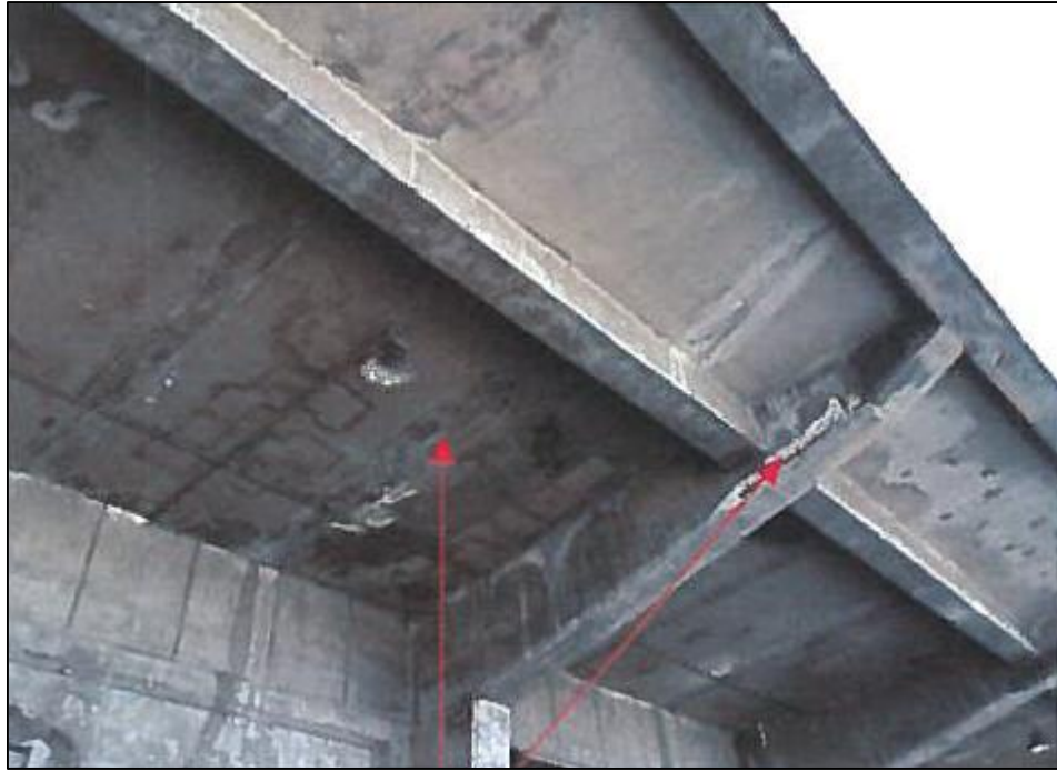
REPAIR SPALLS
