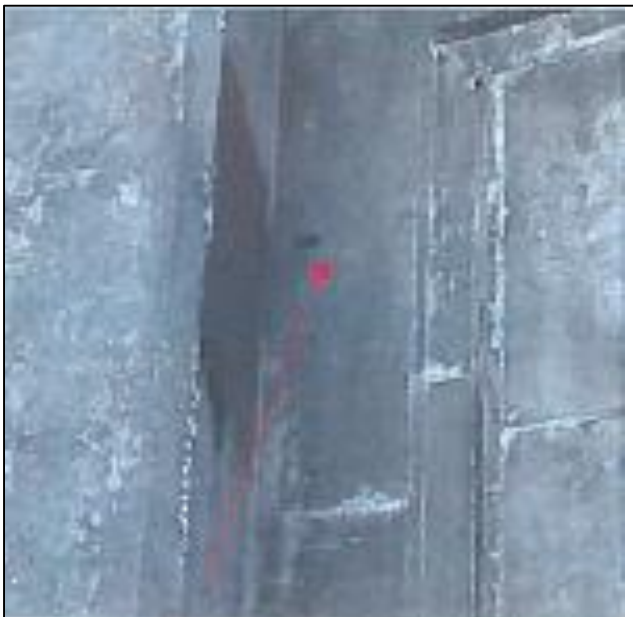
REPAIR SPALL
