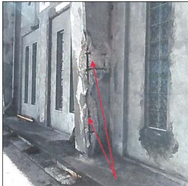
REPAIR SPALLS
