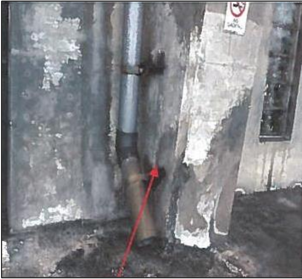
REPAIR SPALL
