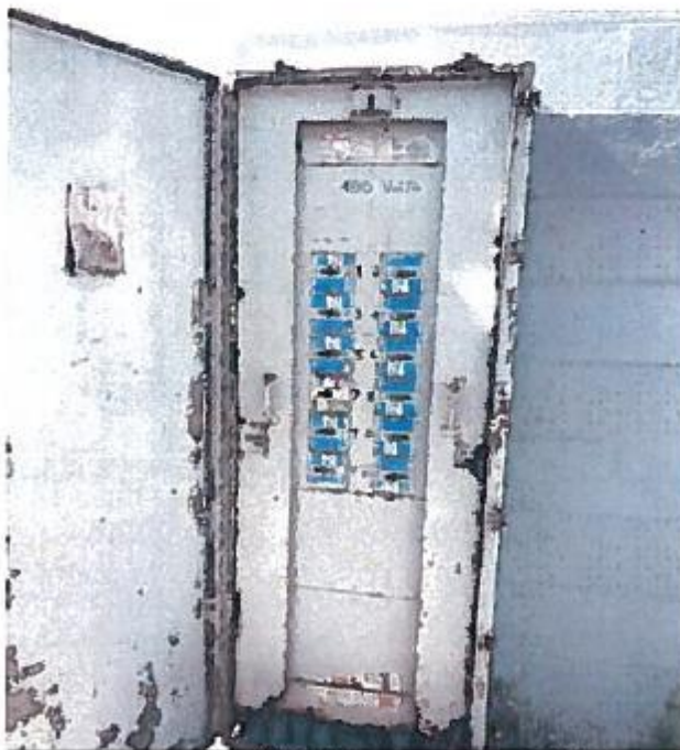
Sub- Panel for 480V and 240 V – 3PH, 4W
