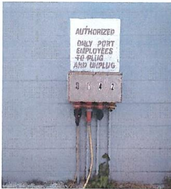
Existing 4 Gang Reefer Outlets 480V/ 3PH/ 32 Amps.
