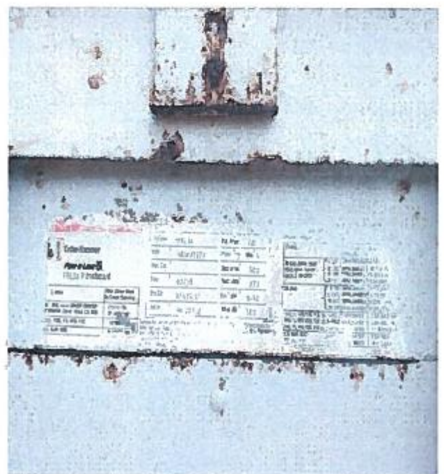
Sub- Panel for 480V and 240 V – 3PH, 4W
