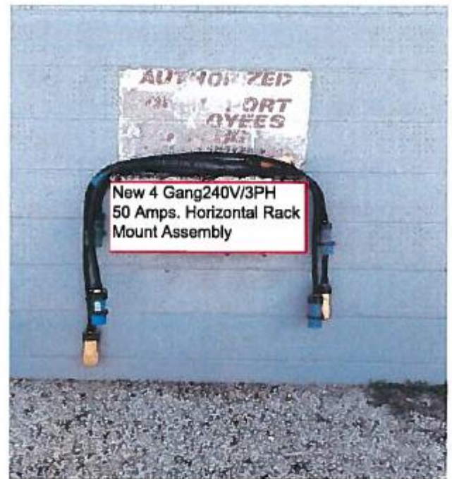
New configuration of 4 Gang 240V/3PH/ 50Amps. Reefer Outlets with safety interlocked outlets and actuator rod.
