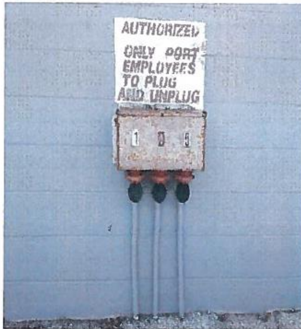
Existing 3 Gang Reefer Outlets 480V/ 3PH/ 32 Amps.
