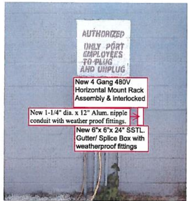
New configuration of 4 Gang Reefer Outlets 480V/ 3PH/32Amps.
