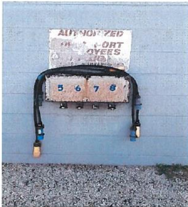
Existing 4 Gang 240V/ 3PH/50Amps. Reefer Outlets
