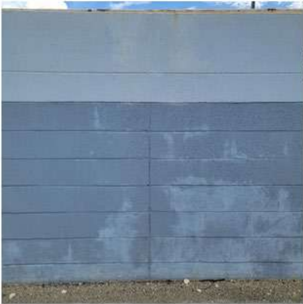
Figure 15 Example of Control Joint
