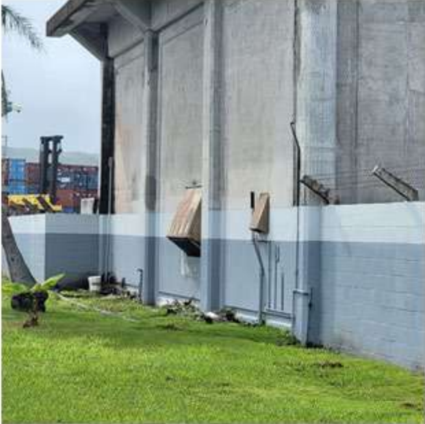
Figure 1 Welding Shop – Wall to be painted
