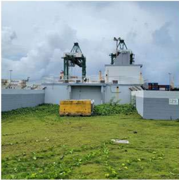
Figure 5 Lower Tower – Wall to Be Painted
