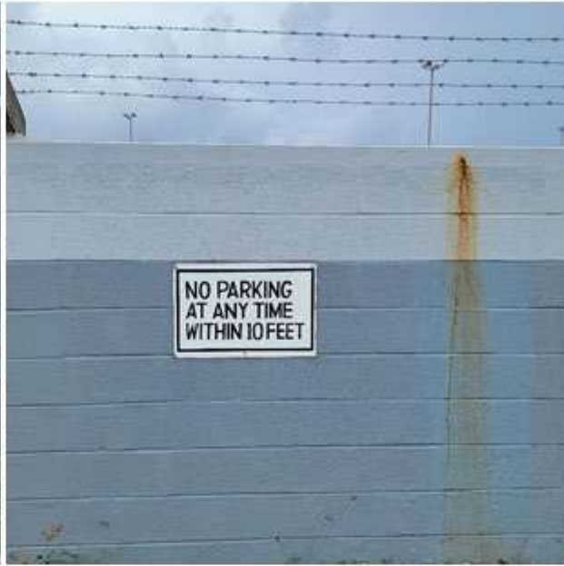
Figure 14 Example of Sign - To Be Removed and Reinstalled. Sizes Vary.
