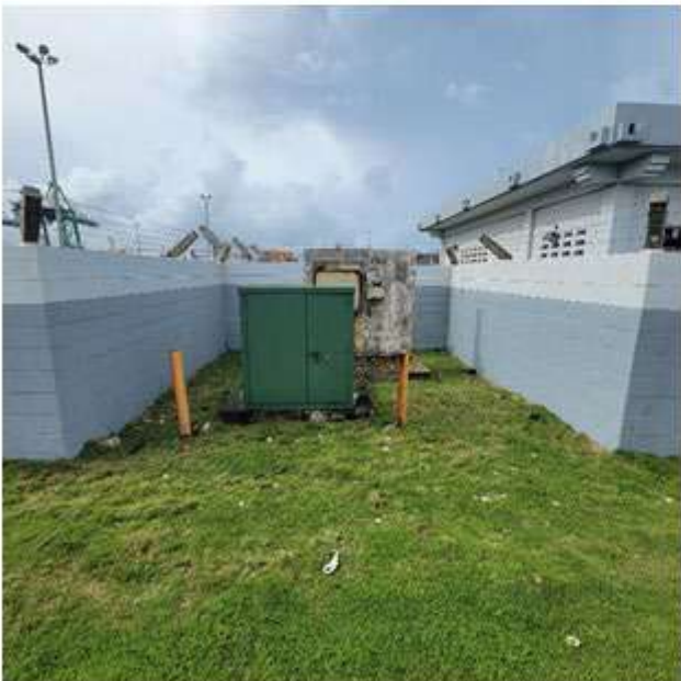
Figure 3 GWA Pump Station Bldg.
