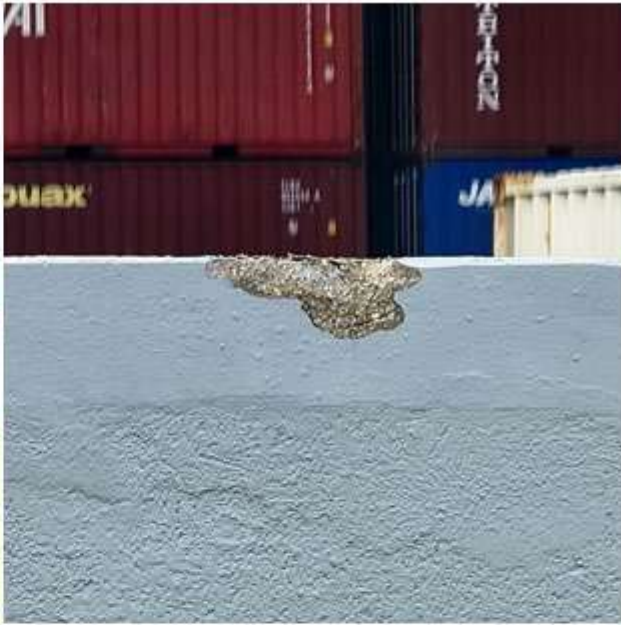
Figure 6 Lower Tower - Wall to Be Painted
