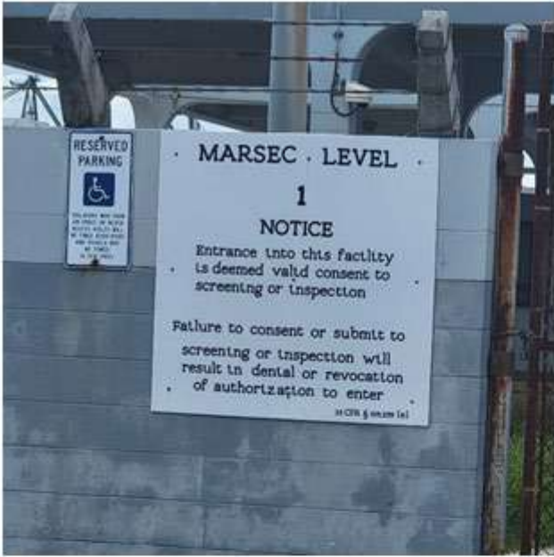
Figure 13 Example of Sign – To Be Removed and Reinstalled. Sizes Vary.
