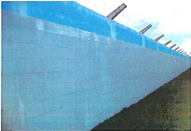
CMU Wall North Side
