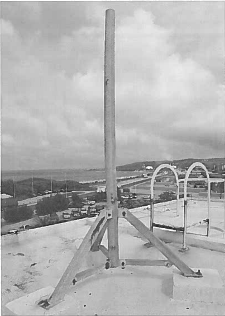
Figure 4: Galvanized Steel Angular Supports Concrete Blocks
