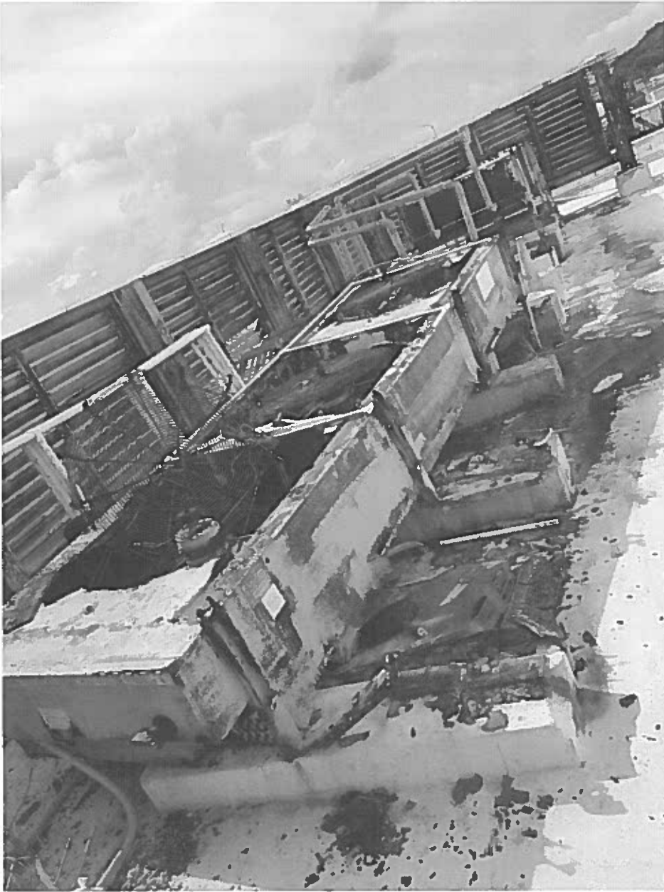
Figure 1: Central AC System
