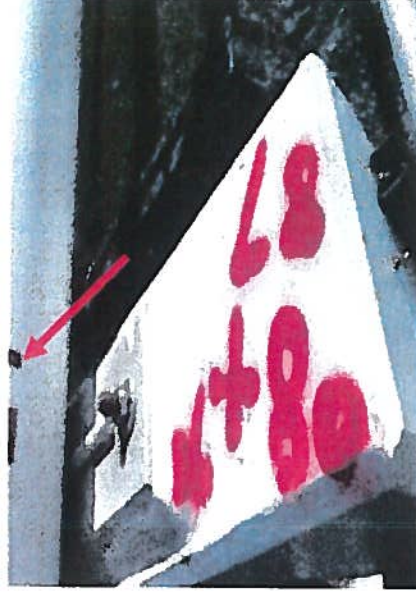
Station 08+47 Corrosion of the Welded Joint of the Unleaded Pipeline
