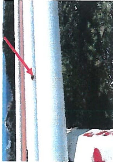
Station 03+33 Corrosion of Unleaded Gasoline Pipeline and Joint.
