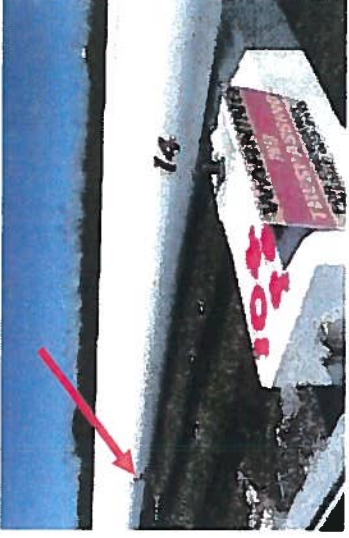
Station 10+94 Corrosion of Unleaded Gasoline Pipeline
