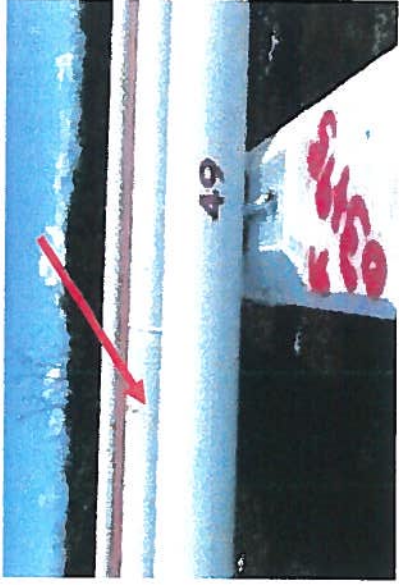
Station 03+95 Corrosion of Jet Fuel Pipeline
