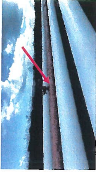
Station 04+04 Corrosion of Fire Salt Waterline Gate Valve & Fire Hose Connection
