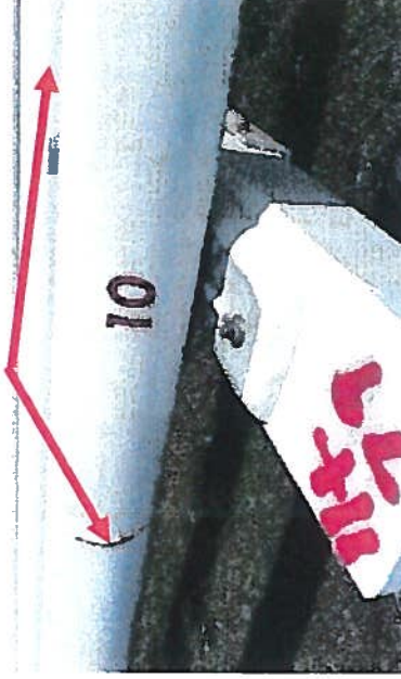
Station 10+94 Corrosion of Unleaded Gasoline Pipeline
