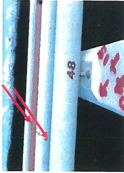
Station 03+95 Corrosion of Jet Fuel Pipeline
