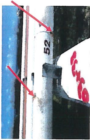
Station 03+33 Corrosion of Unleaded Gasoline Pipeline and Joint.
