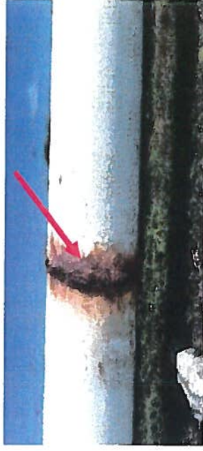
Station 09+29 Corrosion of Welded Joints Unleaded Gasoline Pipeline
