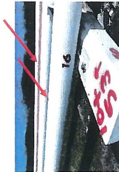
Station 09+96 Corrosion of Fire Salt Waterline and the 2" Dia. Gate Valve/Hose Connection and the Jet Fuel Pipeline,
