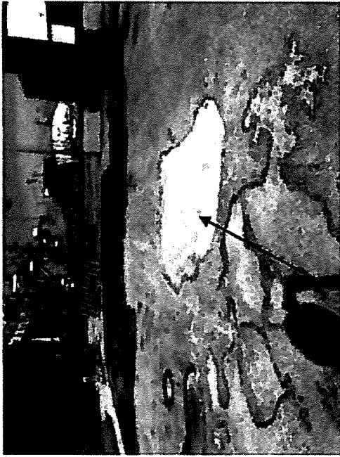
Excavate backfilled Area of Repair = 10' X 10' X 5'
